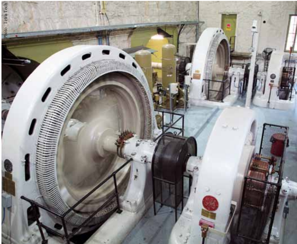
Complete rehabilitation and upgrade of the 2GS hydroelectric power station for Energy Ottawa.
